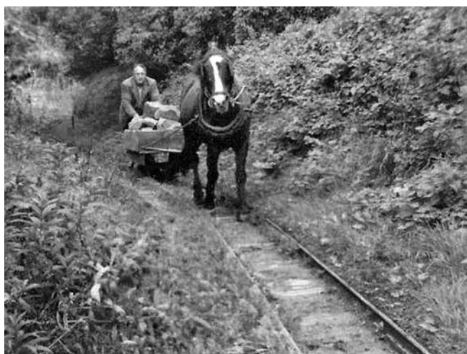
Colley Hill hearthstone mine in 1956. Mined stone is being conveyed to the nearby on site factory by Alfred Turrell and the horse 'Stocking'. The narrow-gauge line has a gradient downwards to the north, into the mine. Photo by Michael Ross
